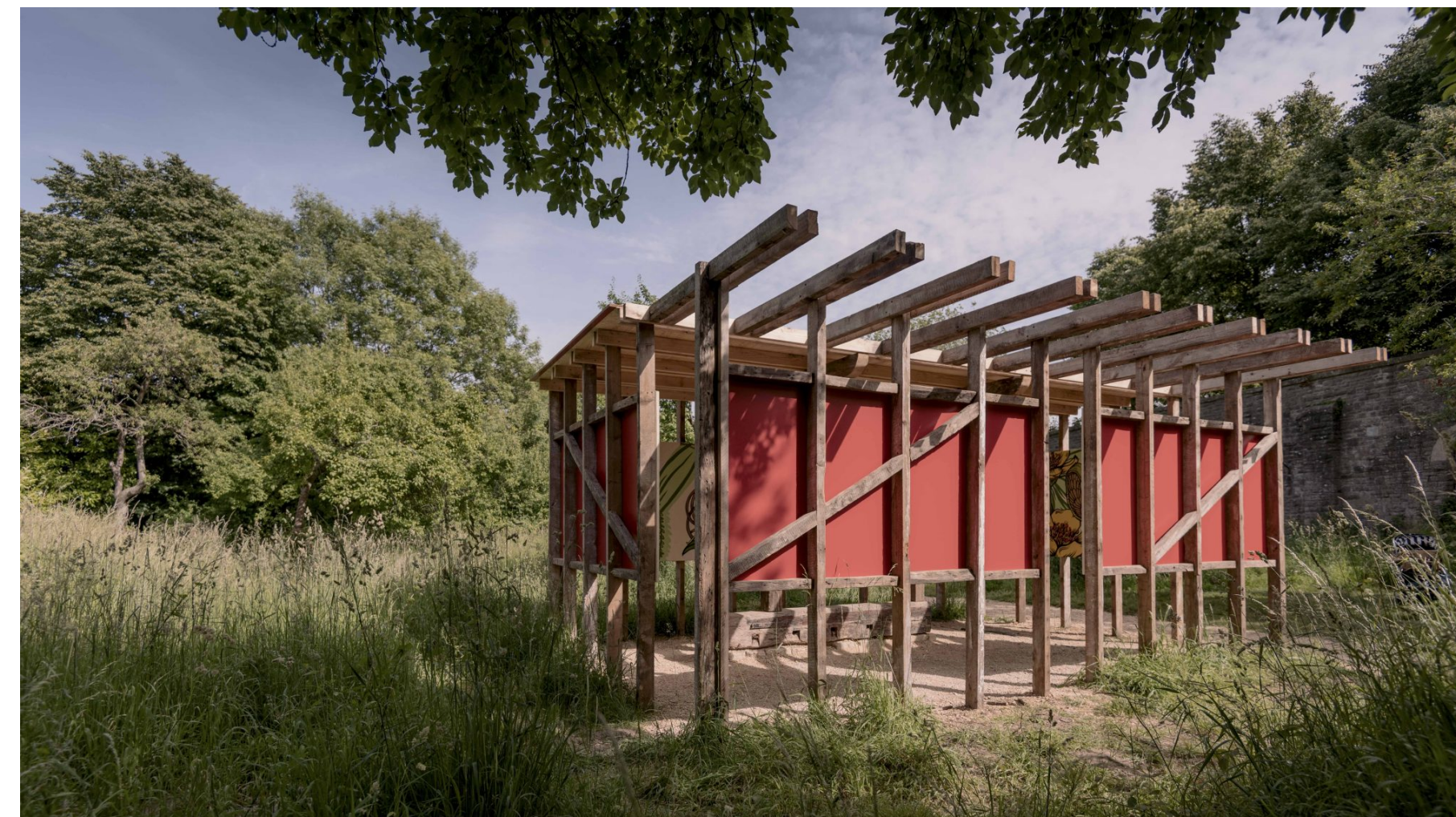
The folly is constructed from materials mined from other decommissioned buildings, in turn it will be deconstructed and reused once the event has finished
