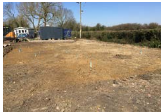
PEGGING OUT The Covid pandemic at the start of 2020 meant building was delayed because of lockdowns.
