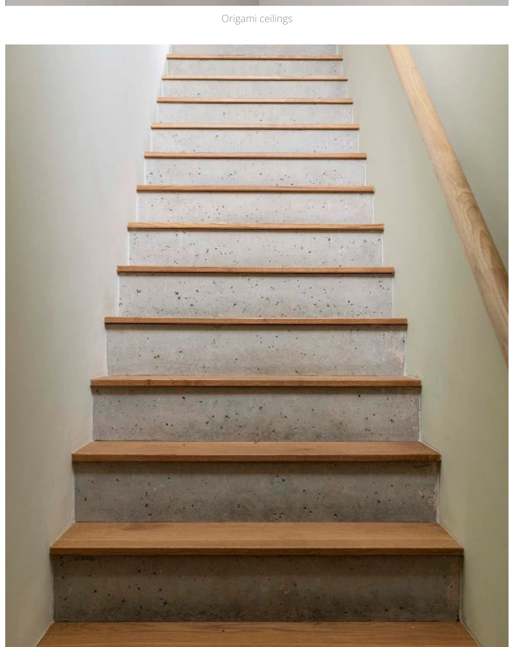
Concrete and Oak Stair
