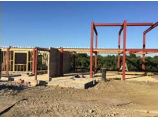
STEEL FRAME Erected in just one day, the property's steel frame underlays the charred timber cladding.
