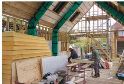
**INSULATION PANELS** 'Boathouse' interior with insulation panels ready to be fitted
