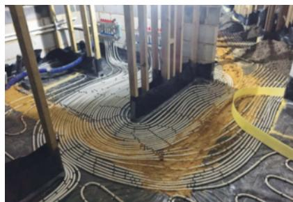
**HEATING PIPEWORK** Installation of pipes that form the underfloor heating
