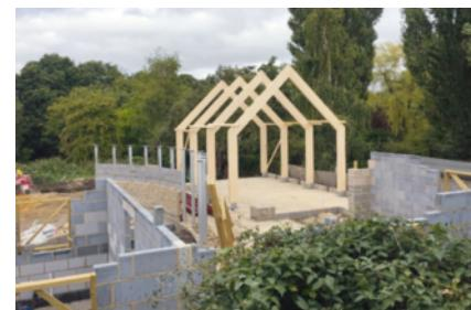
**GLULAM FRAME** Fitting the glulam frame for the section known as the 'boathouse'
